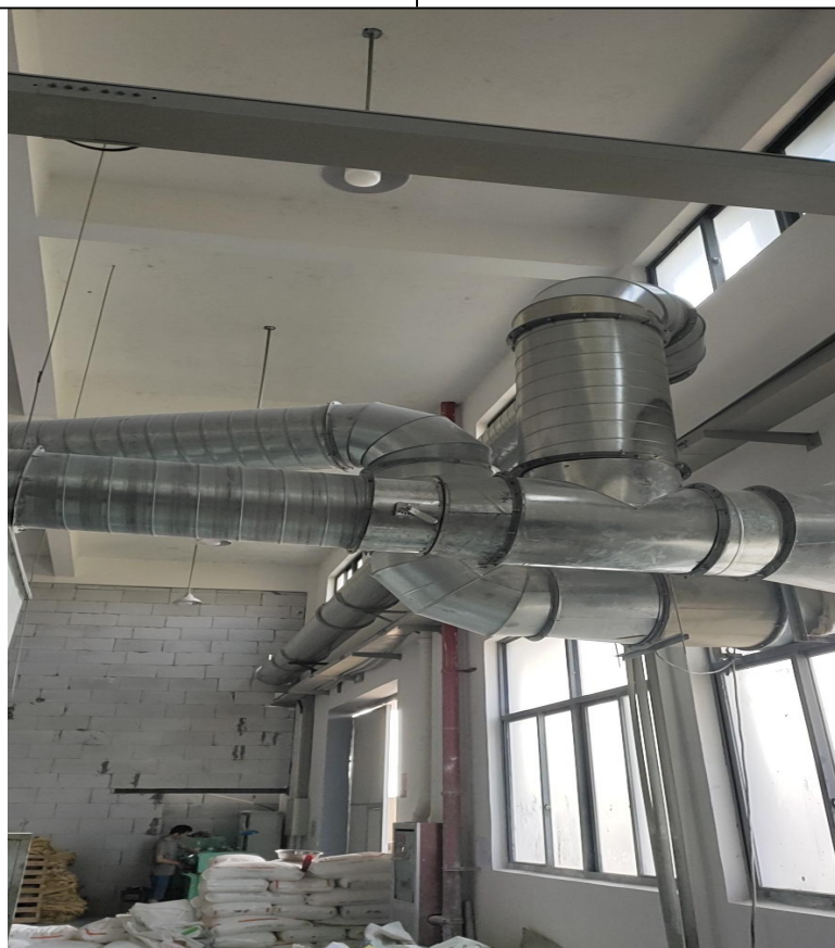
集气罩安装开关阀
